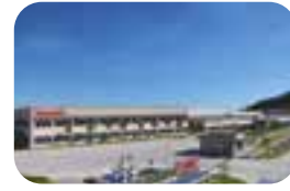
THAILAND Makita Manufacturing (Thailand) Co., Ltd.
